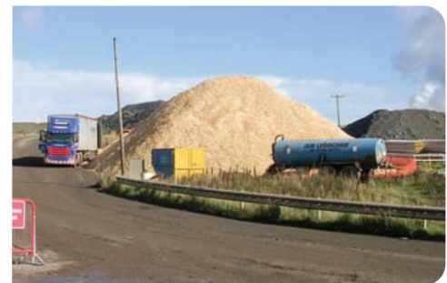
Woodchips being delivered as part of the new bio filters at TEG Environmental Ltd site.
