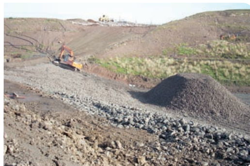
Phase 10 construction work ongoing at Binn Landfill
